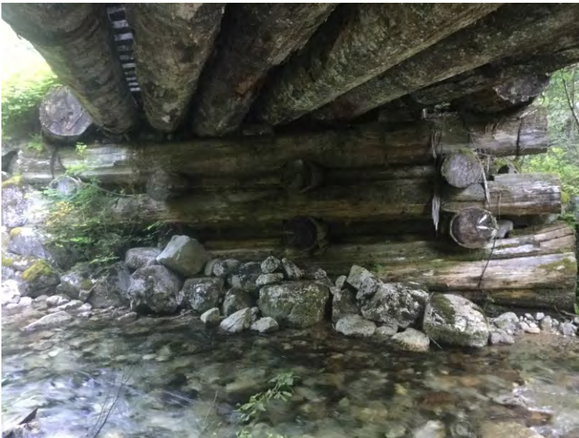
Left Bank Abutment
