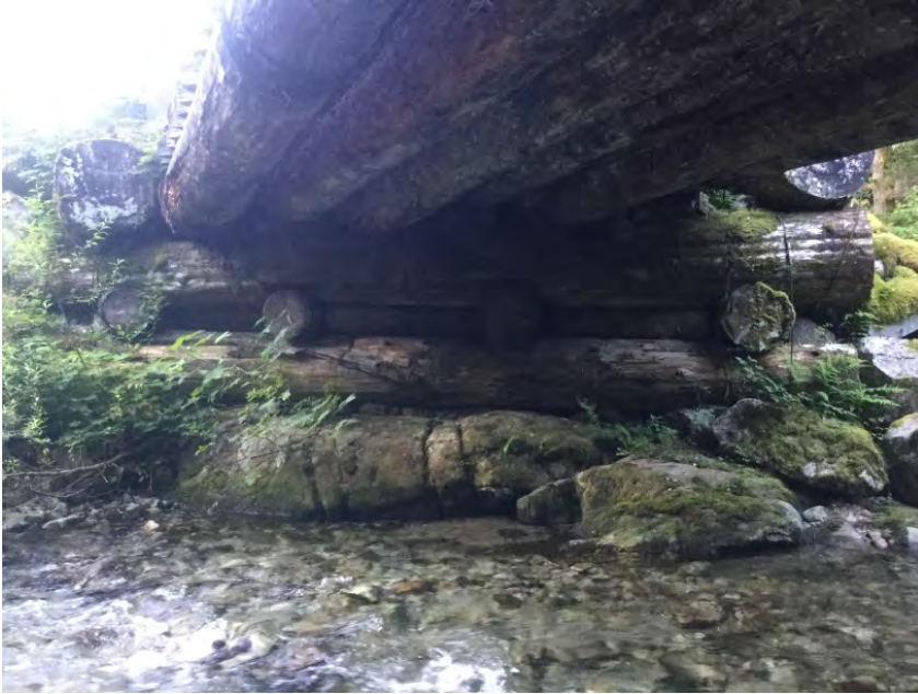
Right Bank Abutment
