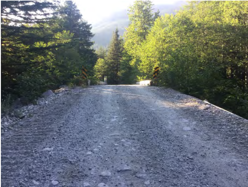
Right Approach Facing Bridge
