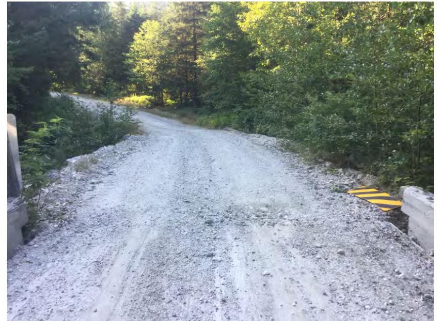
Left Approach Facing Away From Bridge
