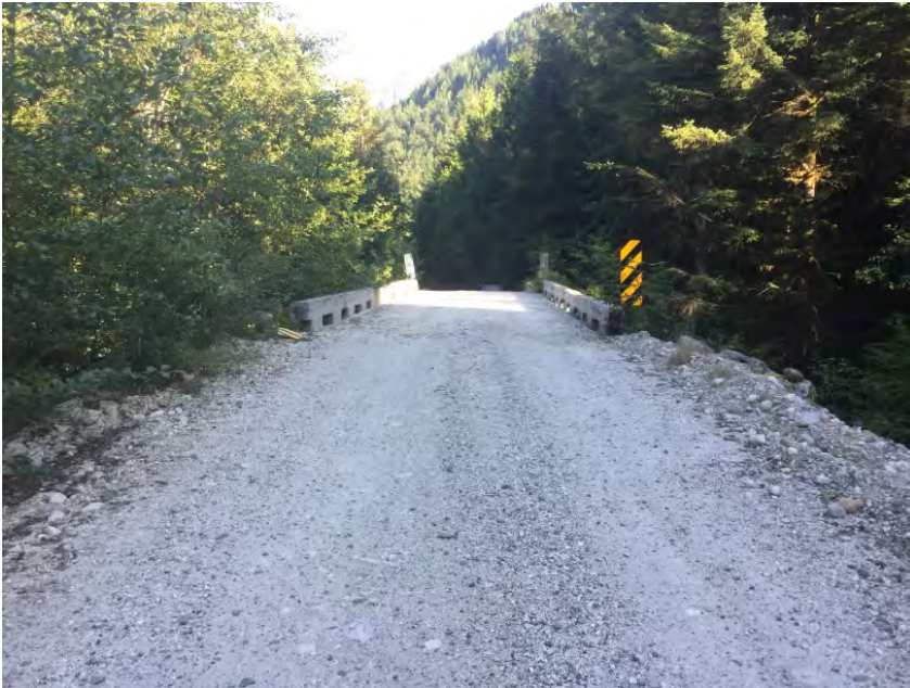
Left Approach Facing Bridge
