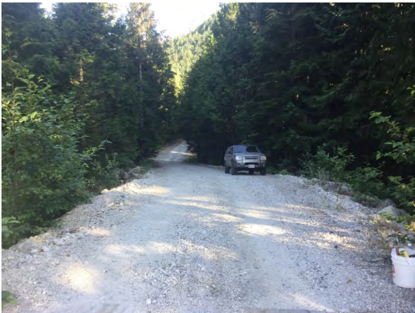
Left Approach Facing Away From Bridge
